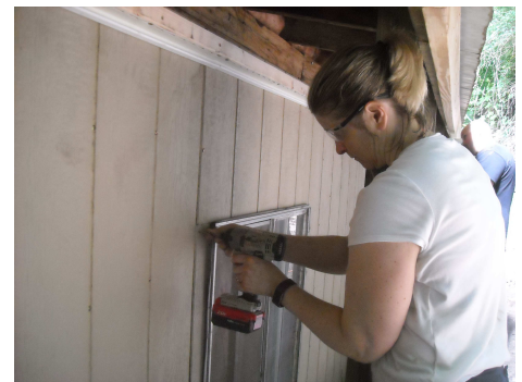
Lori Farrell installs window molding during the 2018 SWAP trip.
