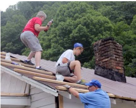
(Left): Lynne, Emily and Mark work at putting on a metal roof for Mr. Tyrone. (Above) Jeff hammers in a board at the top of Tooter's new steps.
